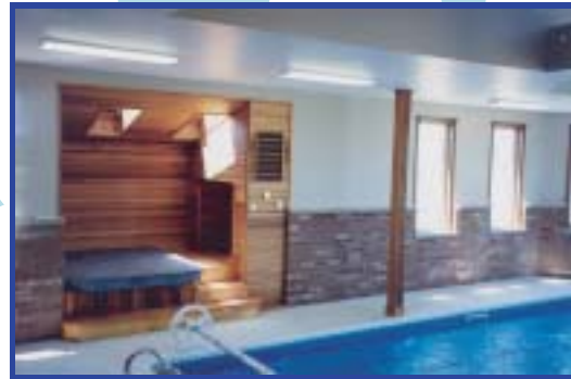
Pool water heating, pool dehumidification, pool air conditioning, pool area heating. Virgil, Ontario
