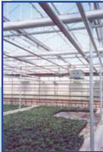
Boiler operation - indoor greenhouses with extremely low CO and CO2. Grimsby, Ontario
