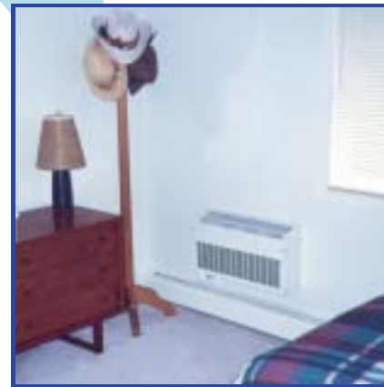
Retrofit wall units. Individual room control from one main outdoor unit. Welland, Ontario
