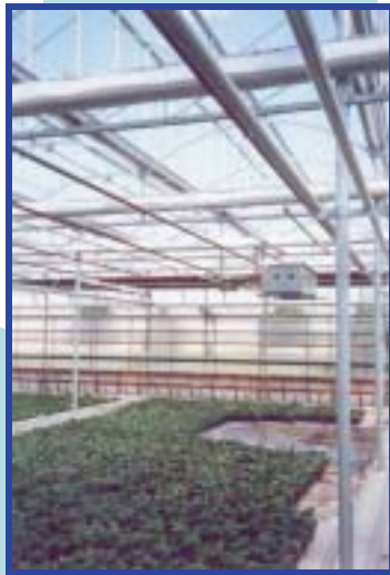
Boiler operation - indoor greenhouses with extremely low CO and CO2. Grimsby, Ontario
